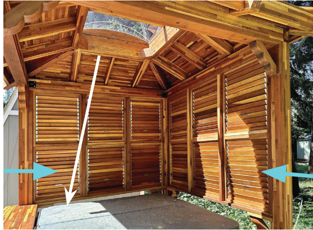
Allow light to pass mainly from above and allow an angled roof and leveled access to determine how it hits
