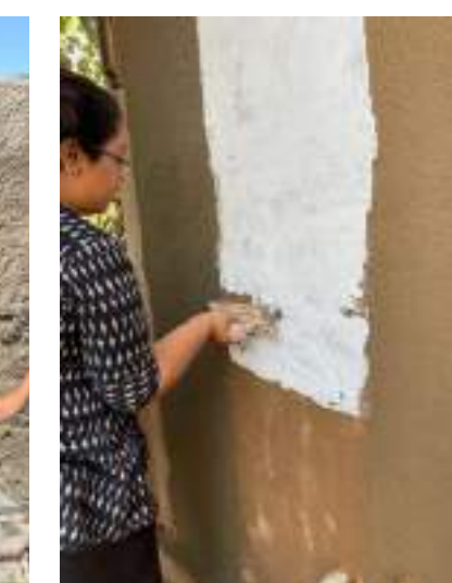
Process: Finishing coat of Mud Plaster (Group Work)
