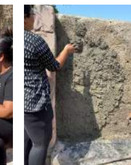
Process: First coat of Mud Plaster (Group Work)
