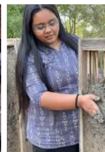
Process: Wattle and Daub wall (Group Work)
