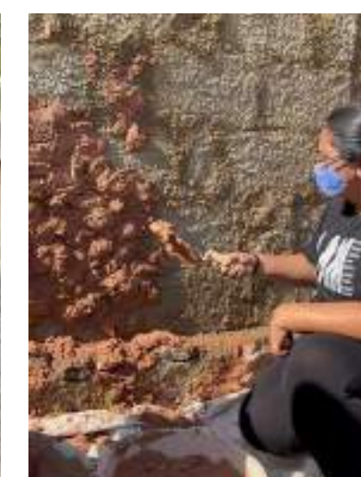
Process: First coat of Lime - Surkhi Plaster (Group Work)
