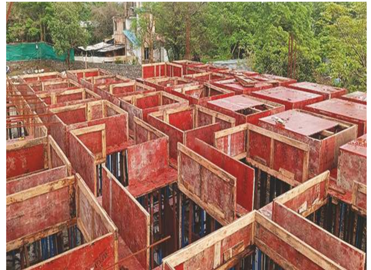
Framing and reinforcement procedures
